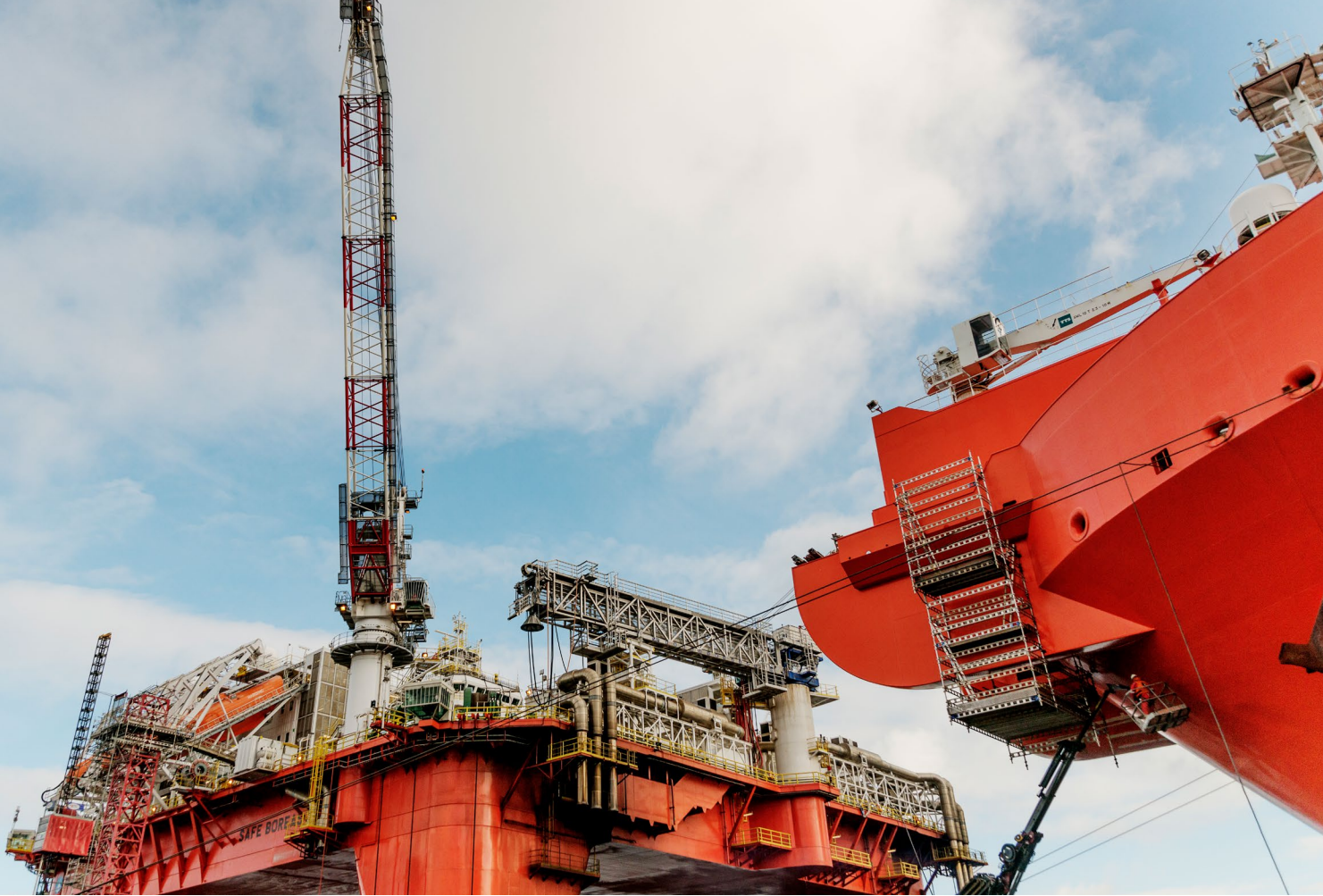
Photo: Pictures from the rig Safe Boreas while docked in Mekjarvik outside of Stavanger. Credit: Tommy Ellingsen / the Norwegian Oil and Gas Association from Offshore Norge via Flickr.
